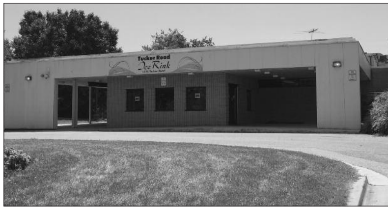
PHOTOGRAPH COURTESY OF MARYLAND DEPT OF NATURAL RESOURCES Former Tucker Road Ice Skating Center
