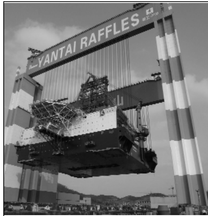
CREDIT: WIKIPEDIA/HAAKMAN Finding significant off-shore oil reserves could turn Cuba into an oil exporter, possibly even thawing relations with a still oil-hungry U.S. Pictured: The Scarabeo 9 oil rig while still under construction in China in 2009. It is now 30 miles off of Cuba's coast and just 60 miles south of the Florida Keys.
